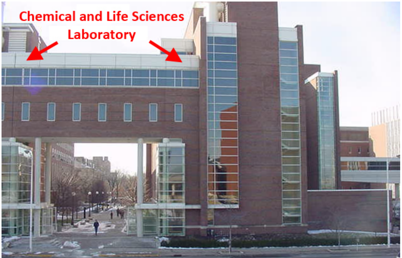
West view of the north building of the Chemical and Life Sciences Laboratory (CLSL), the main entrance for the School of Molecular and Cellular Biology (MCB), including the Department of Microbiology.
